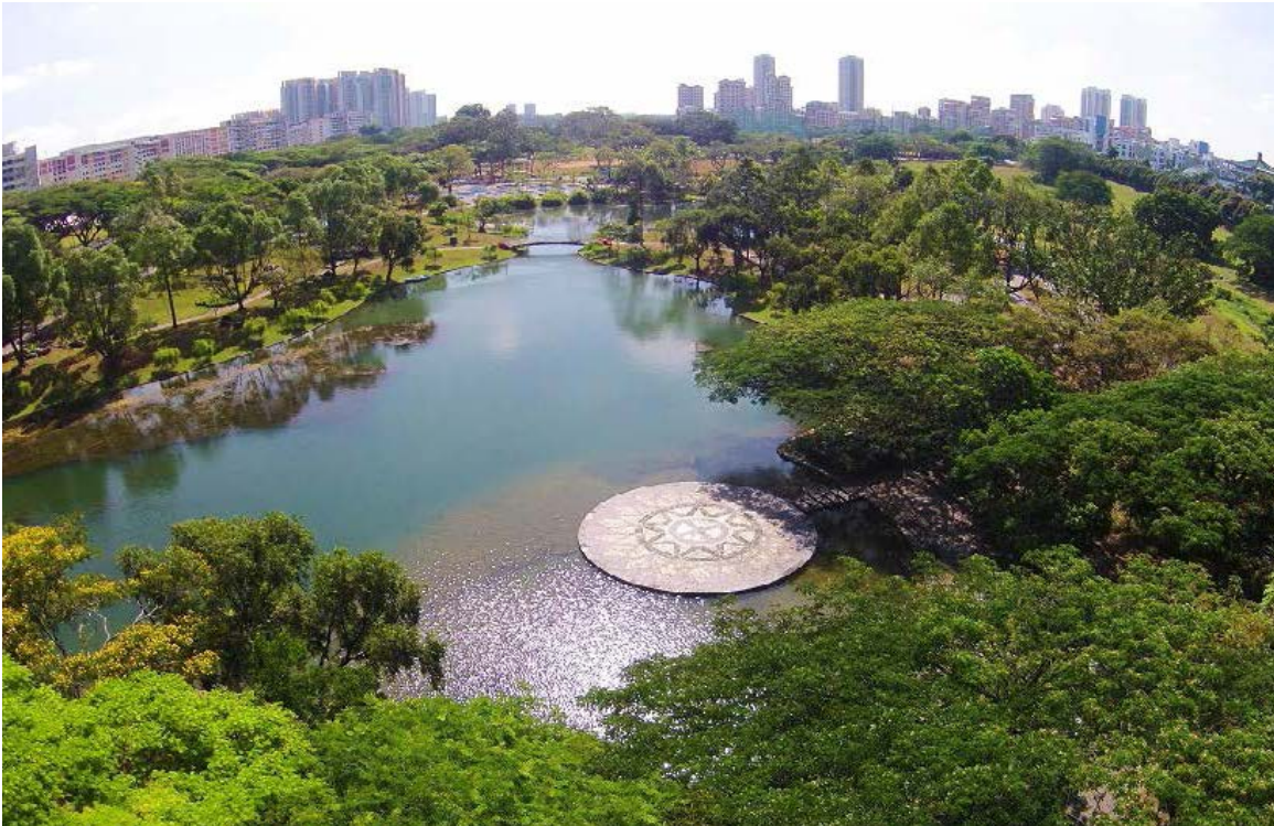
A naturalised restored stream that used to be a concrete drain runs through the Bishan-Ang Mo Kio Park. As a drain, it used to serve the sole function of flood control but with the restoration of this section of the Kallang River, this freshwater ecosystem now provides numerous ecosystem services like drought amelioration, flood mitigation, recreation, education, biodiversity conservation, etc. This popular park in Singapore is home to otters, over 100 species of birds, 40 species of dragonflies and damselflies, more than 50 species of butterflies and moths, more than 10 species of native riverine plants, etc. © National Parks Board
