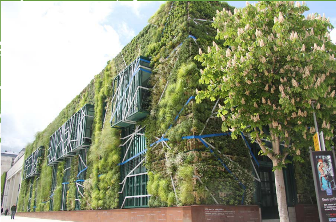
The eye-catching green facade decorates the European Congress Centre in Vitoria-Gasteiz, Spain. © Quinta fotógrafos
